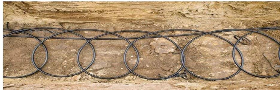
Ground source heat pumps can be an efficient way of using electricity to heat your church, by capturing and boosting heat drawn from underground.
